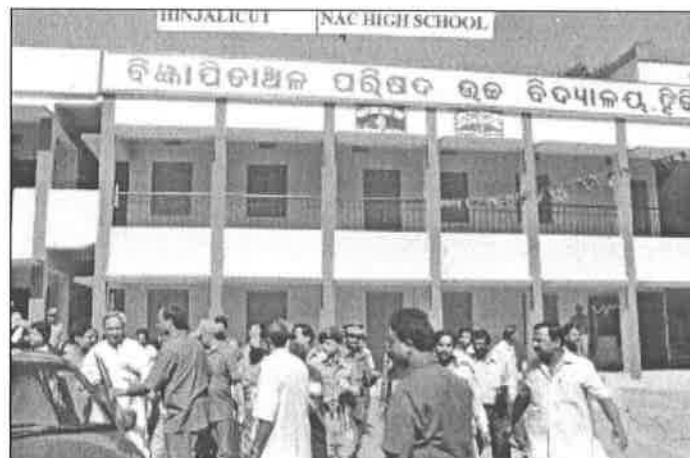
NAC High School, Hinjicut built with MPLADS (Lok Sabha) Funds
