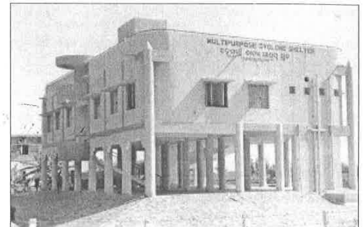
Multipurpose Cyclone Shelter
