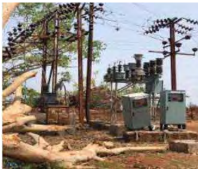
Figure 6.1: Damaged 33 kV Panel and Substation
