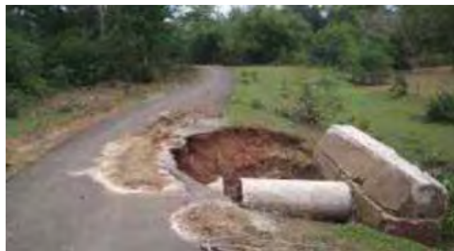
Culvert/embankment damages
