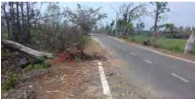
Tree uprooting and damages to berms
